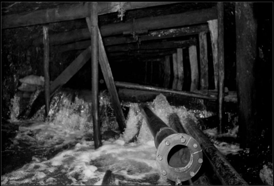
This picture was taken at the Hebe coalmine near Collie in south-western WA in 1965, after an aquifer that overlay the coal seam was accidentally breached. The flooded mine never reopened. With few exceptions, methane-rich coal seams lie below the regional water table and are permeable.
